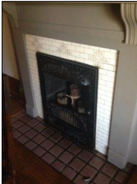
10. Coal-burning fireplace - not in service
